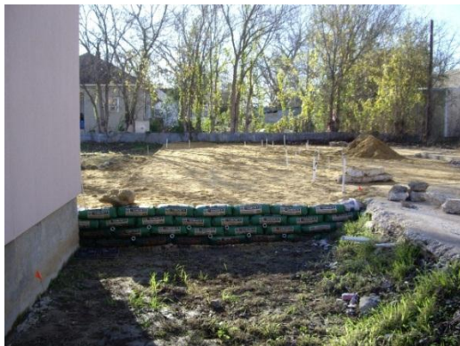
Fill dirt in place
