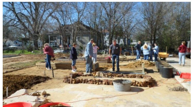
Laying the Rock Bed
