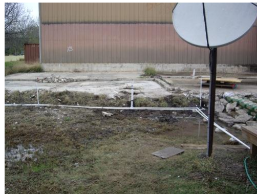
Irrigation Line installed
