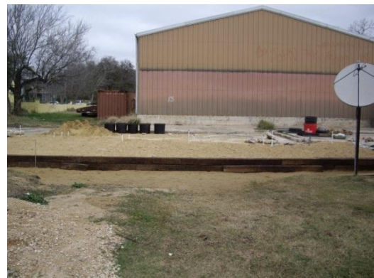
Front retaining wall
